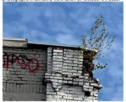
Bricks are missing and the remaining ones, at an angle they are not meant to be. The mortar is significantly compromised, as reflected by the fact that vegetation is growing out of the corner of the building.<sup>1</sup>
