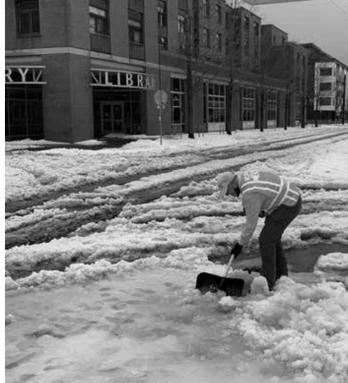
NET member Chris Blumenthal clears a storm drain on Tillamook.
